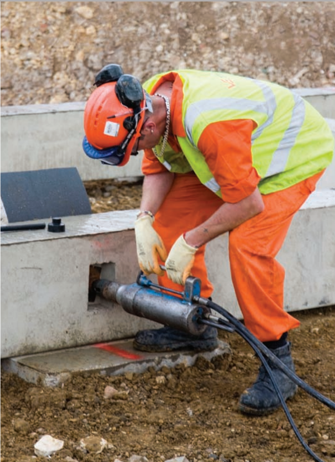
LEFT Van Elle Smartfoot System: the post tensioning operation in progress
