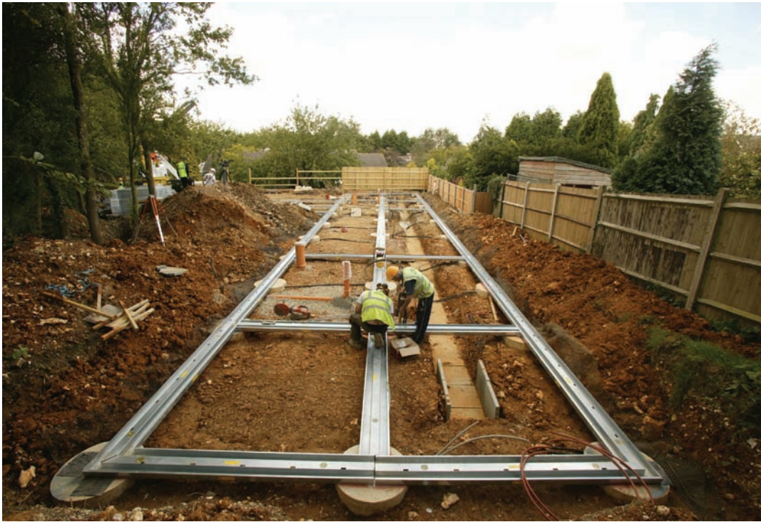
ABOVE Roger Bullivant's SystemFirst galvanised sections installed on piled supports
