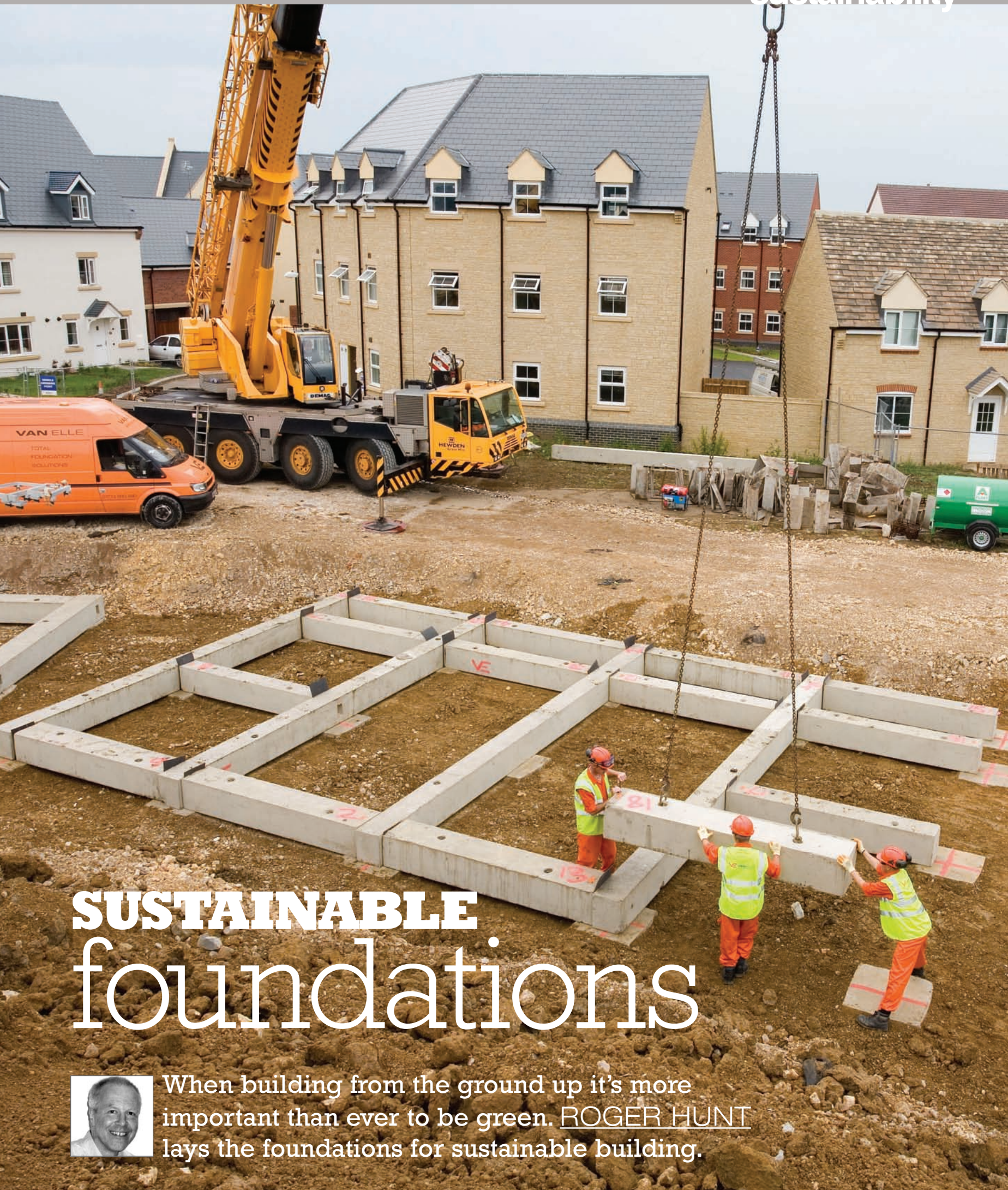
ABOVE Van Elle Smartfoot System: the Smartfoot beams being lowered into position
