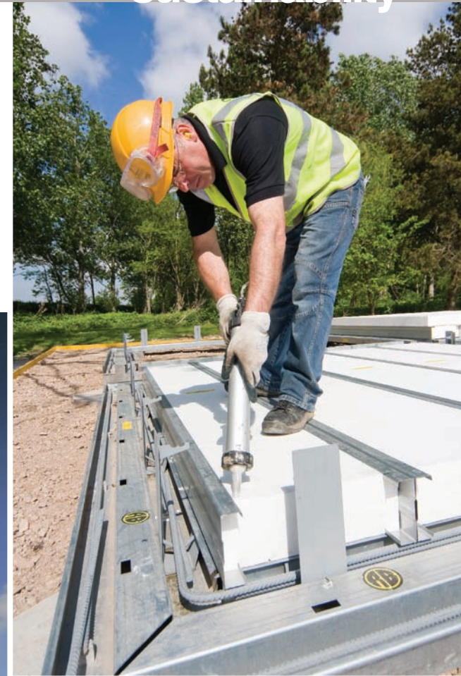
RIGHT Roger Bullivant's SystemFirst is installed on site. The polystyrene insulation for the floor fits into the galvanised steel frame
